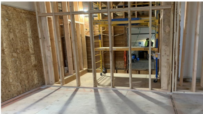
Elevator Shaft Framing
