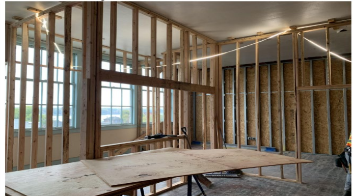
Level 2 Framing at County Counsel 202
