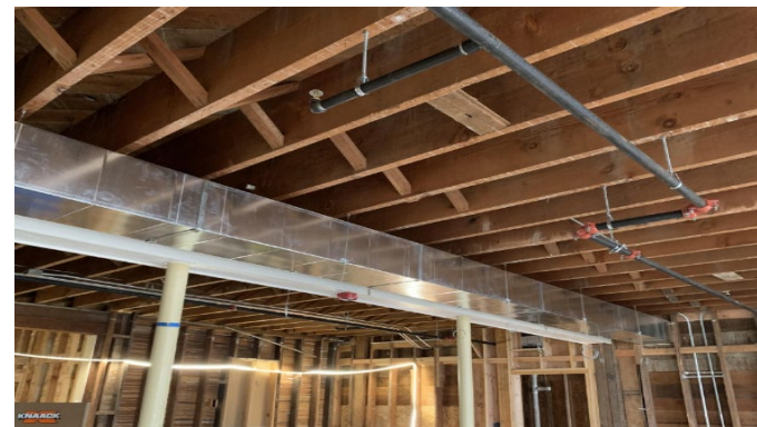
Basement HVAC and Fire Sprinkler Rough-in
